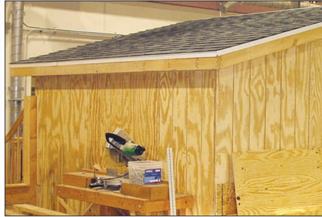
Figure 3: The kiln roof system was designed for outdoor use.
