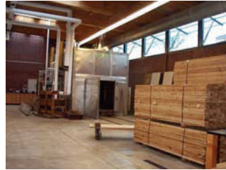
Research kiln for lumber drying.
