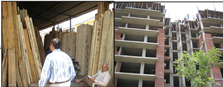
Typical retail outlet for shuttering (left) and shuttering used in construction of a multi-story concrete building (right).
