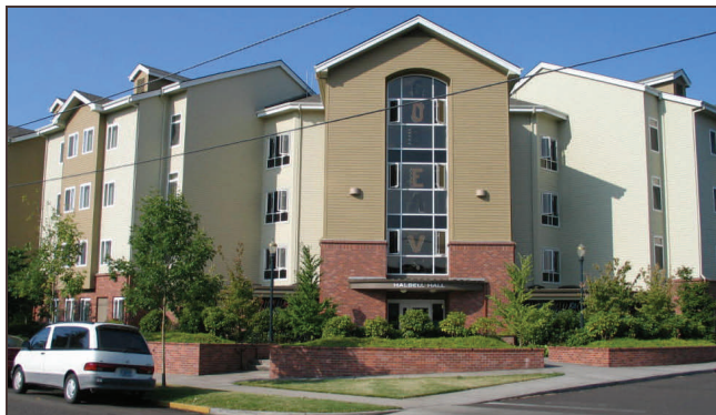
OSU student dorm built in 2002—a 77,000 ft. 2 , four-story, wood-framed and -sheathed building; built faster and at less cost than a concrete-constructed dorm. Selecting wood reduced the use of fossil fuels, used a renewable-sustainable resource, and lessened impact on global warming.
